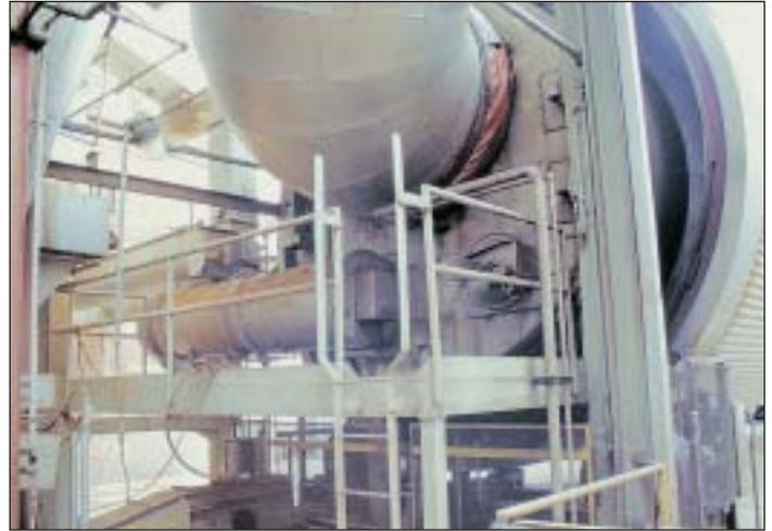
Mixer feeds prepared 65% solids material into rotary drum dryer, below larger duct bringing in process steam.
