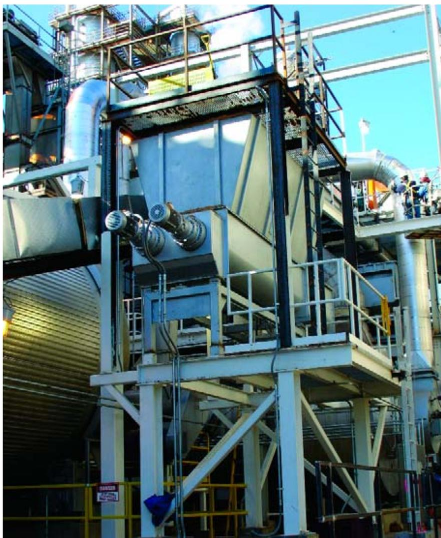
*This dosing bin with twin-screw discharge meters the grain solids into a screw conveyor for transfer to a paddle mixer at the dryer's outlet.*
