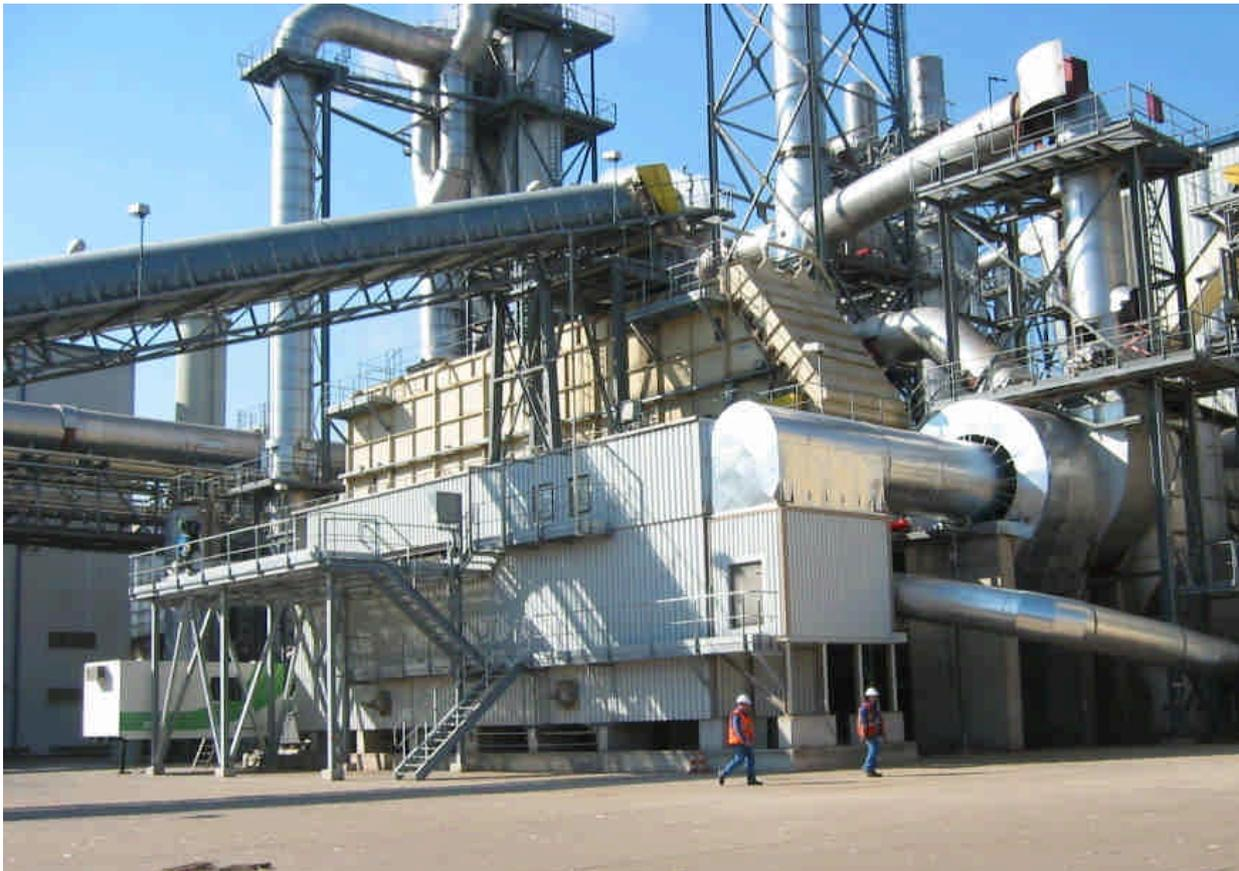
Single pass 5,4 x 24 NH after retrofit to *ecoDry*. In front the heat exchanger. Picture below shows hot flue gas ducting from furnace in the back through the no more used mixing chamber to the heat exchanger
